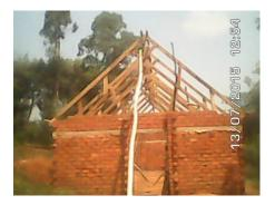
This will be the first church in the Eglise Catholique Anglicane du Congo to be constructed from 'brique cuite' – brick that has been fired in a kiln, and so can withstand heavy rains. As the photographs show, the roof frame is built: now we need money for the roofoing sheets! They cost approximately \$15 - \$20 per 4' x 8' sheet.
